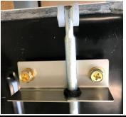
4E - While squeezing the bracket tight around bushing tighten the 2 bracket screws. Repeat this process for the second bracket.
